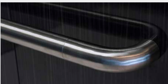
Handrail — round, return end
